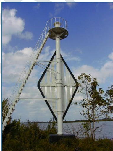
Figure 2 Front leading light with daymark lattice design
