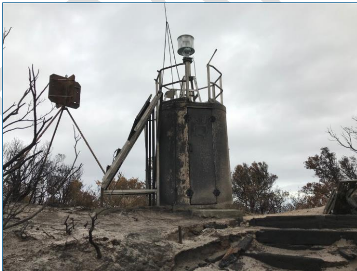
Figure 19 Example of AtoN destroyed by fire
