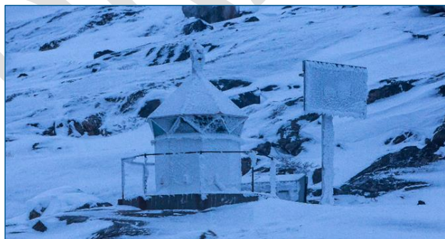
Figure 11 Example of ice on AtoN structure
